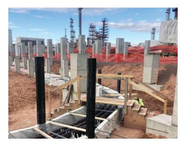
92,000 pounds to 164,000 pounds, and when all were set in place, bolted together and welded to the piers, it formed a building 40 feet wide by 180 feet long and 10 feet above grade. Working together to plan the lifts with our Ironworker Superintendent AJ Westby and Vic's Site Superintendent Mark Brouwer allowed the setting to go flawlessly and ahead of schedule. This new PDC will provide all the electrical for the entire plant when fully operational.
