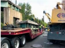
the concrete deck was done to expose the structural steel on both ends, and torches were used to slice through the steel, which was resting on concrete columns. Once this was accomplished, the lift could be made. The father-son team of Steve Levine, shop manager, and Jake Levine, crane operator, lifted and turned the 56-ton section smoothly to the ground parallel to the highway at precisely 7 a.m.
