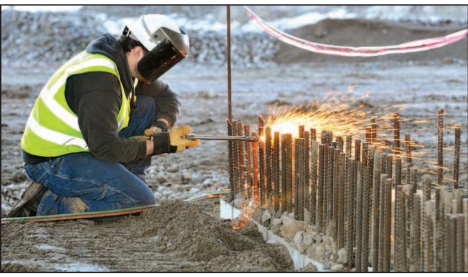
Rebar is cut to length in the crusher plant being built at the Essar Steel site.
