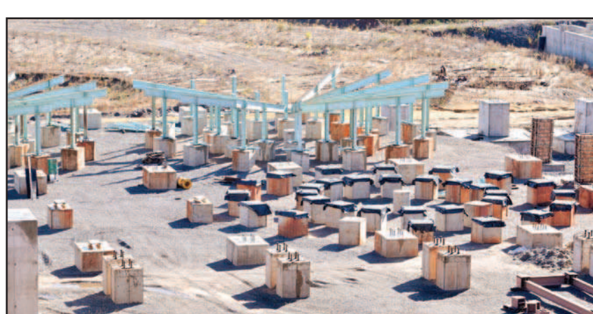
Building materials are laid out mapping where the new facilities will be.
