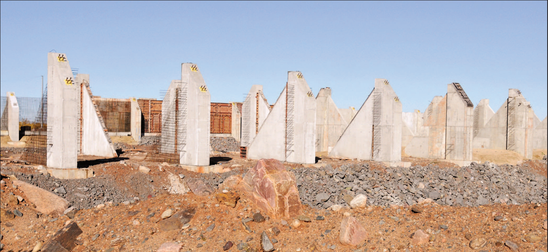
One of numerous buildings under construction at Essar Steel sits on top of a hill.
