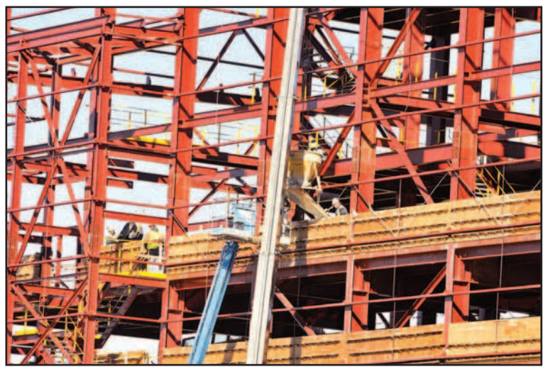
Building crews are moving into full swing with steel and concrete work.
