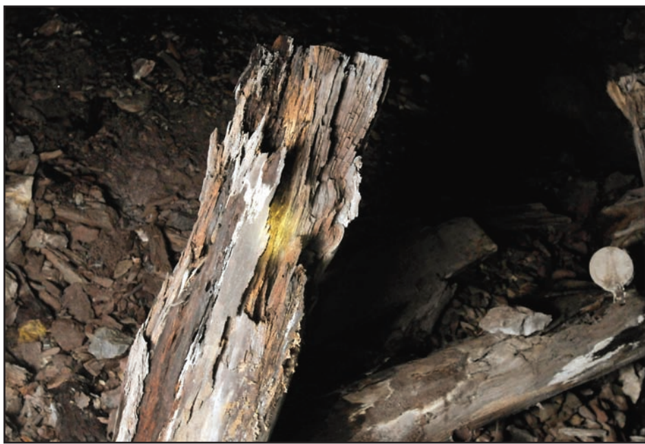
The passage of time and water show in some off-limits areas of the Soudan Underground Mine.
