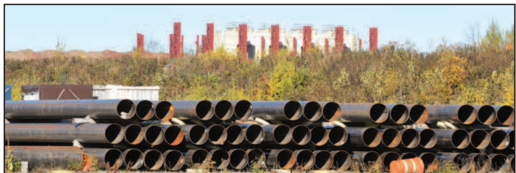
Materials are on location and work is starting to progress at Essar Steel.
