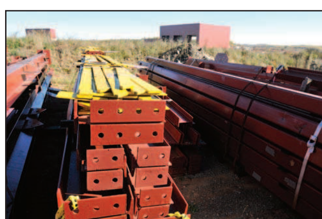
Piles of steel construction material is laid out in strategic locations around the Essar Steel site waiting to be assembled.
