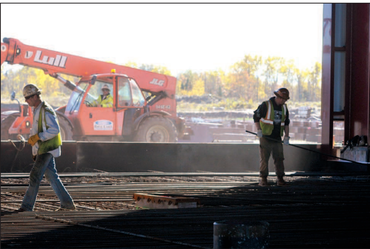
Rebar for the foundation of the crushing plant at Essar Steel are laid into place.
