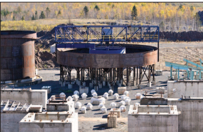
Essar Steel in Nashwauk is still in the early stages of construction, but work is expected to pick up rapidly.
