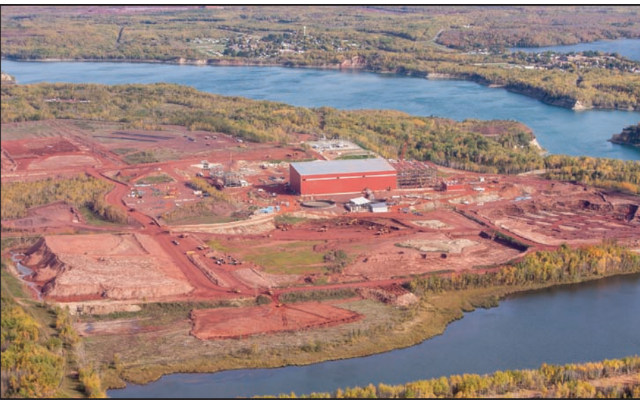
©2014 DAVE WITT/AERO-ENVIRONMENTAL CONSULTING LLC Construction at the new Magnetation plant.
