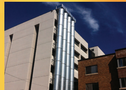
◆ Temporary Fresh Air Ductwork installation
