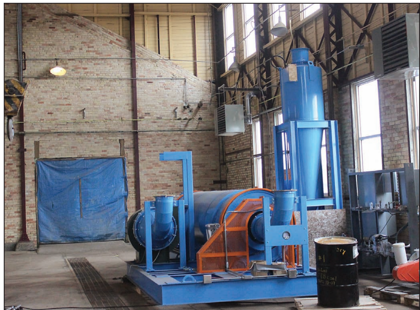
The lab is currently under construction renewable energy building sits in what used to be a train station for U.S. Steel. When completed in the first quarter of 2015, the facility's giant kiln will burn biomass.
