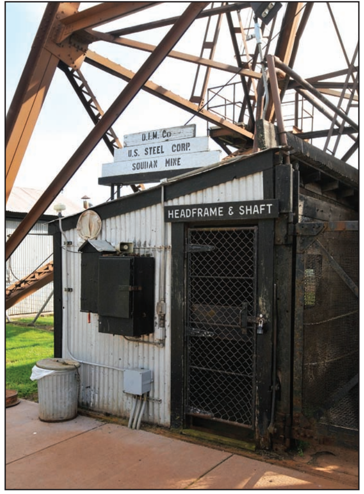
More than 30,000 visitors a year use the same equipment to get to the Soudan Underground Mine as the workers did when the mine was in operation.
