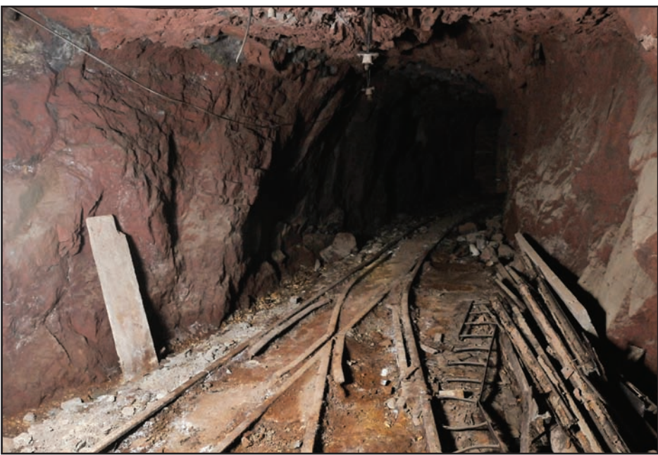
Rusting rail tracks on level 25 stretch into the darkness.
