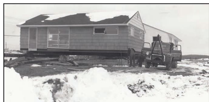
Houses pre-made in Biwabik are trucked in and set on foundations in Babbitt in the 1950s.
