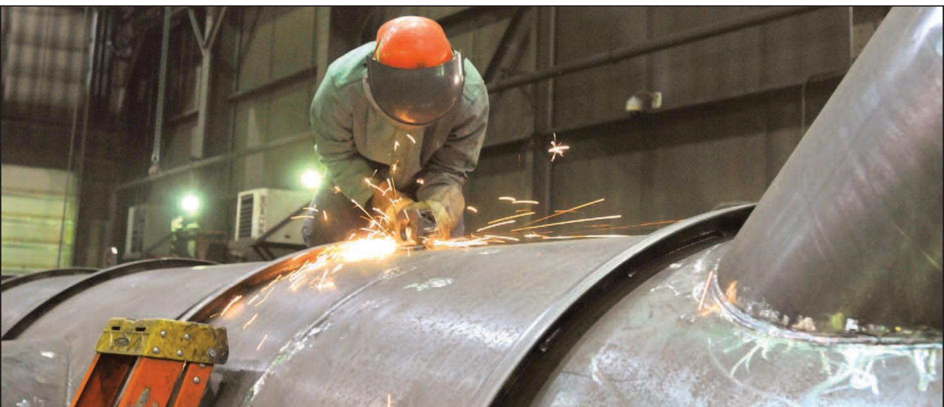
A worker cleans a welded joint on an exhaust stack section.
