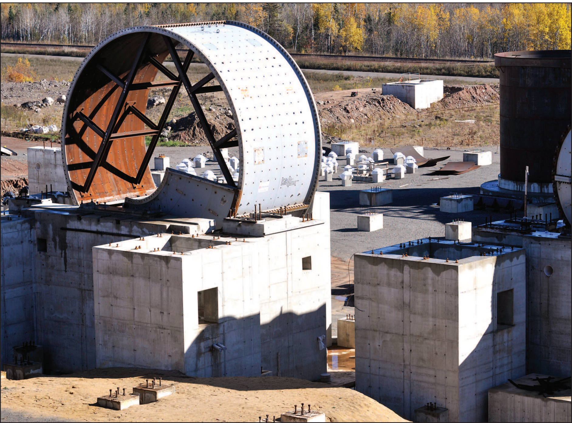
The Essar plant is being built from the ground up.
