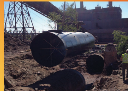
◆ Mill Water Line Replacement
