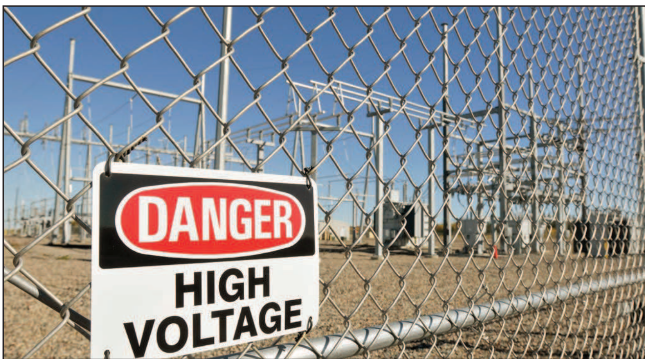
One of two Minnesota Power substations which will be used to power the Essar site in Nashauk.
