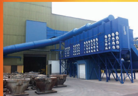
◆ Dust Collection System
