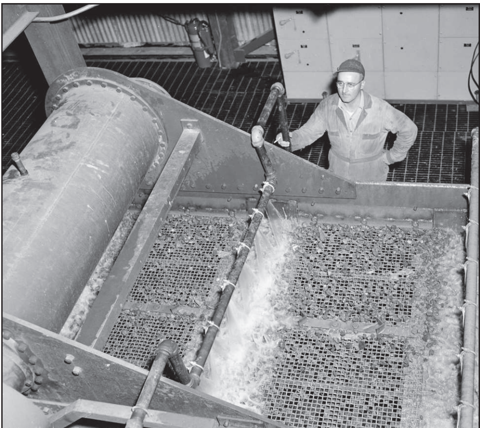
From the June 9, 1955, Herald-Review: The crude ore goes through several sizes of screens to sort out that which must be crushed further before processing. In this picture, Freeman Hane inspects ore going through the secondary screening equipment.
