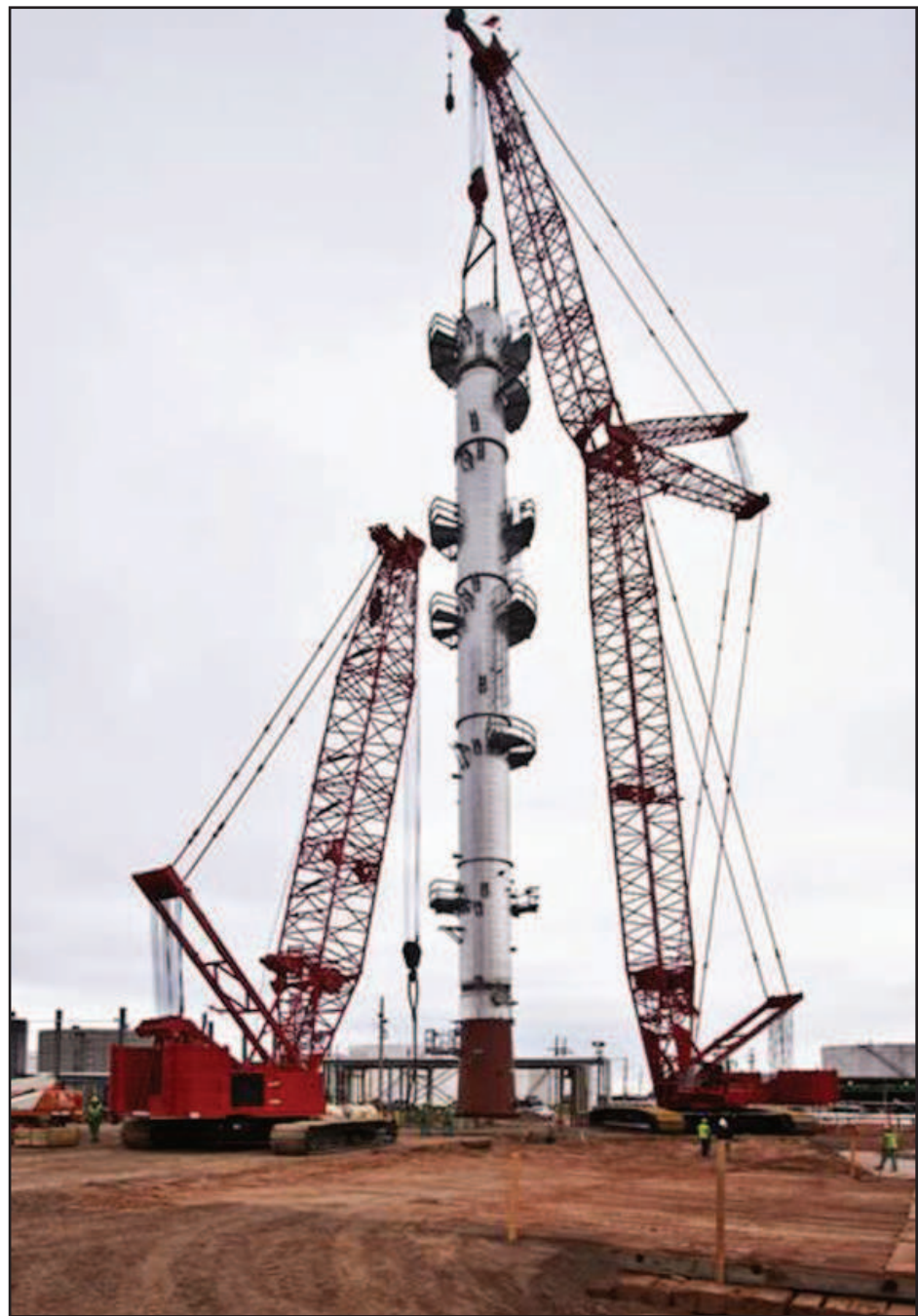
LCI completing a tandem lift of an oil refining vessel utilizing a 16000 Manitowoc crane with a luffing jib, and a 14000 Manitowoc tailing crane.
