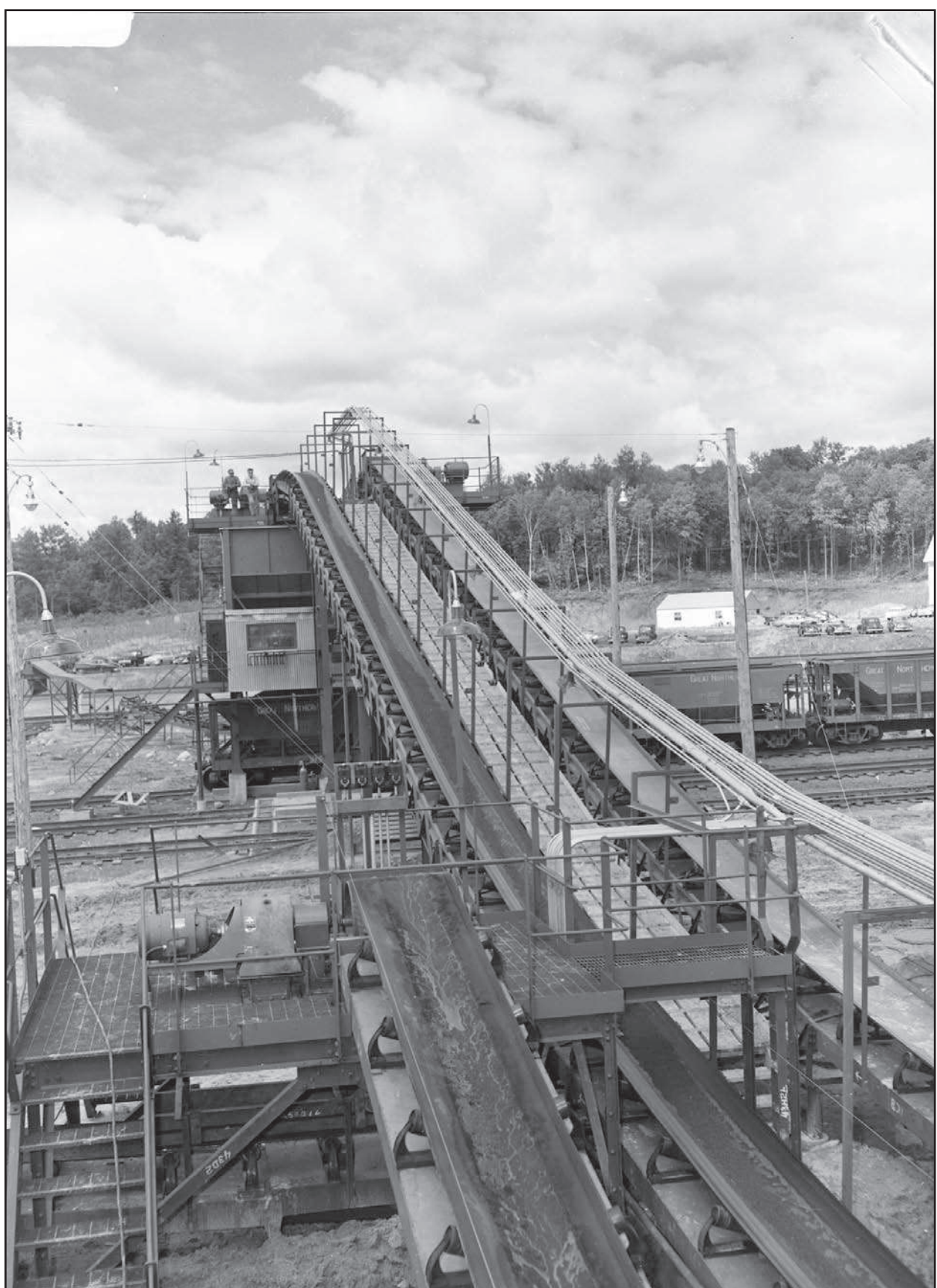
From the June 9, 1955, Herald-Review: After treatment of the ore is completed, it is carried by conveyor belts to a pocket from which it is loaded into railroad cars. A stacker and loader are being assembled beyond the new loading pocket which will be used to stockpile ore when not loading into railroad cars. Conveyor belts are also used to carry the tailings away from the plant.
