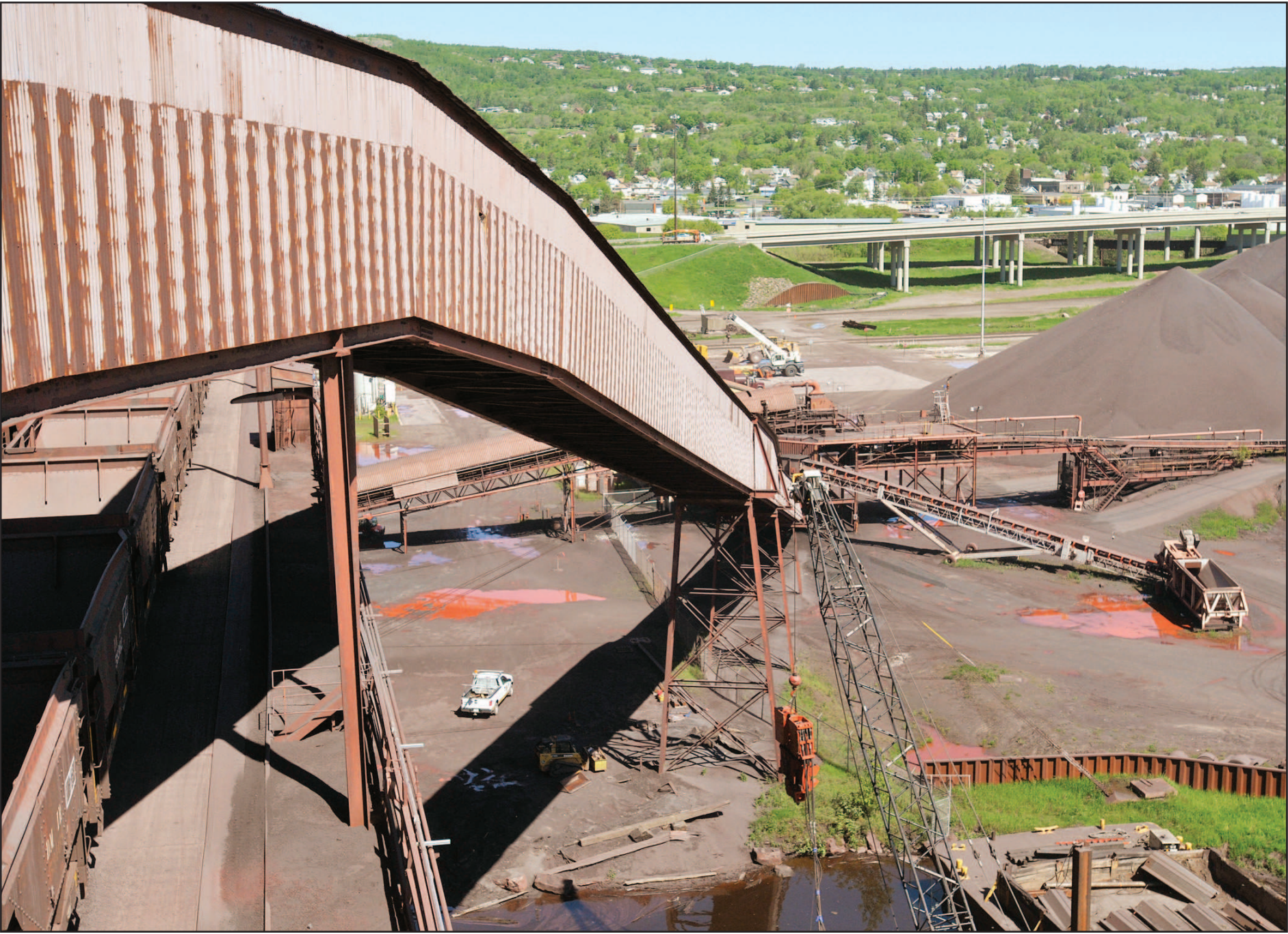
A conveyor system brings ore from stock piles to the loading dock.
