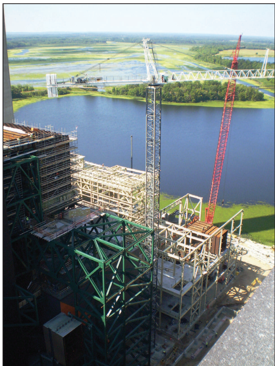
LCI erecting steel and setting equipment at a northern Minnesota power plant utilizing a Terex Peiner SK575 tower crane and a Manitowoc 999 crawler crane.
