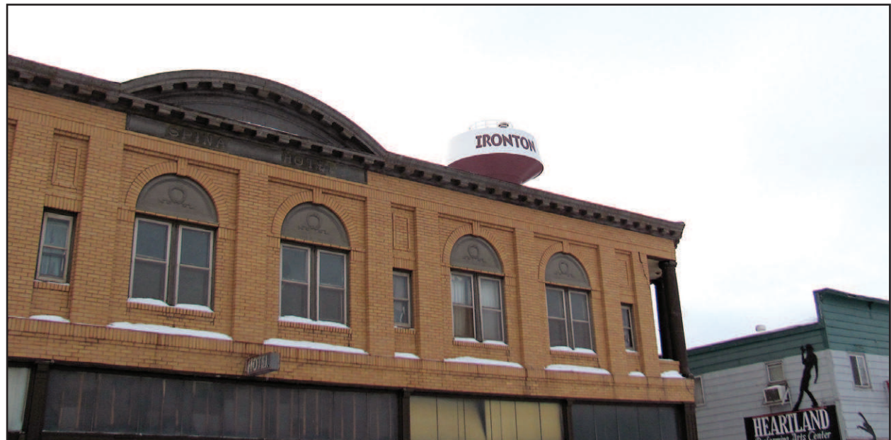
The Ironton water tower peeks from behind the old Spina Hotel in Ironton.
