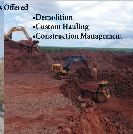
Essar Steel Minnesota Tailings Basin
