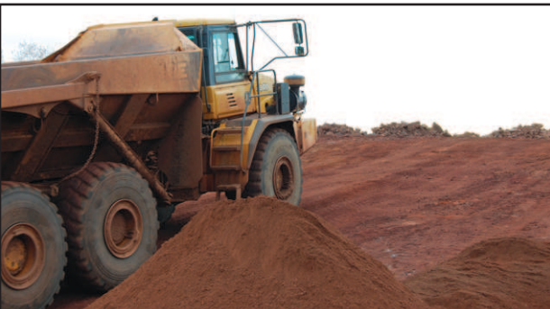
A Hammerlund crew brings heavy equipment into a construction site.
