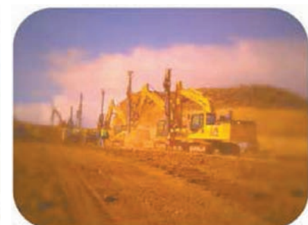
Ruby Pipeline Drilling and Blasting
