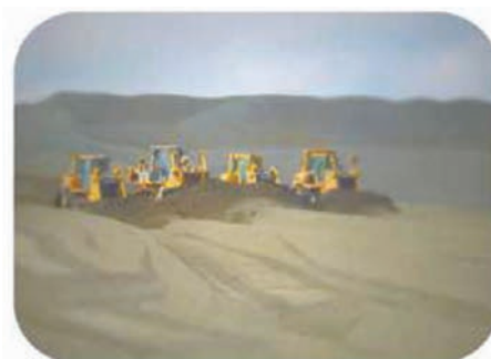
Quade Dozer Push, at United Taconite
