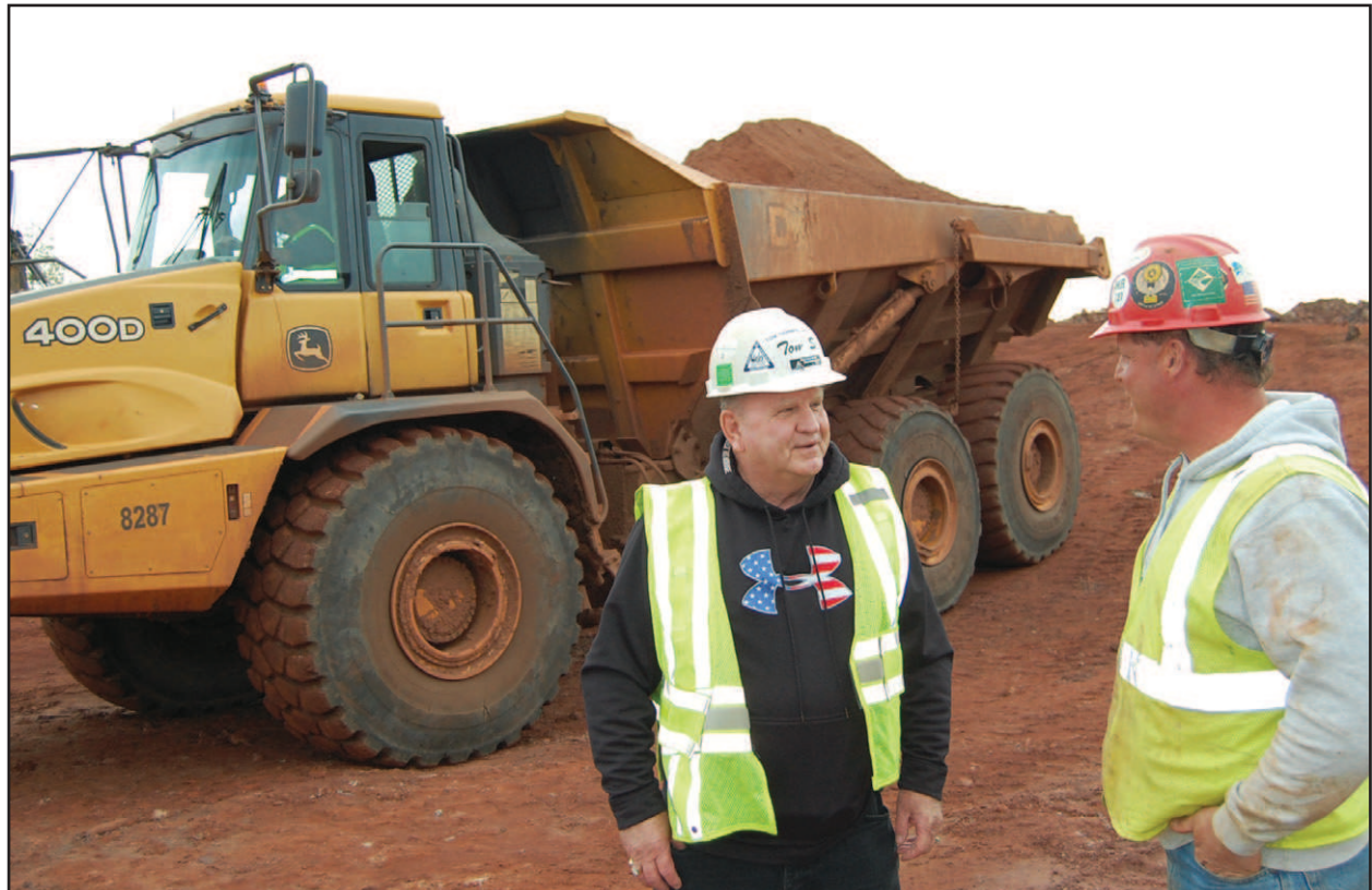
Tom Hammerlund, Sr., (left) talks with Hammerlund Construction grading superintendent Jodi Neary on a site for Essar Steel Minnesota.
