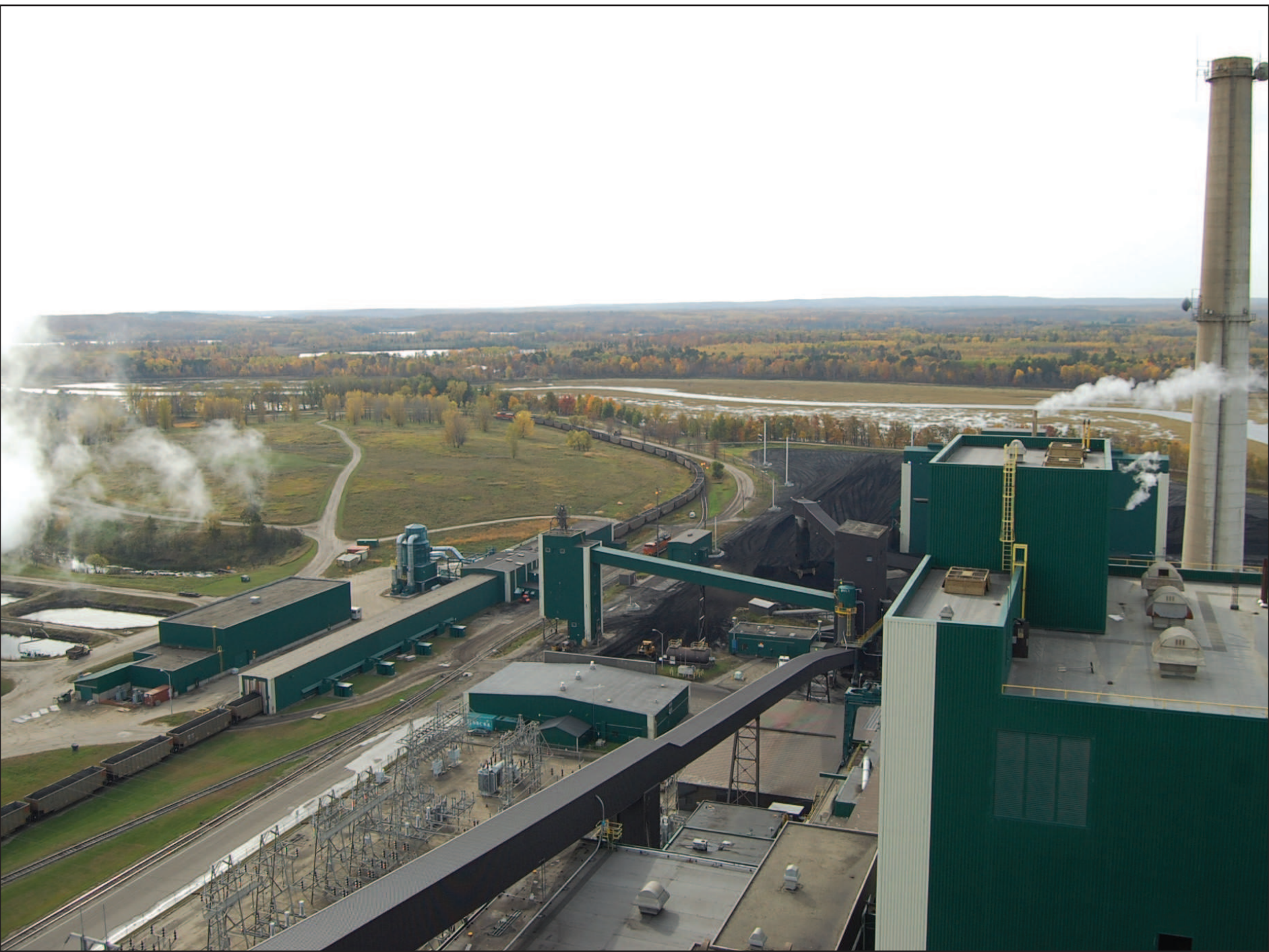
The Boswell Energy Center in Cohasset generates power used by area mines.
