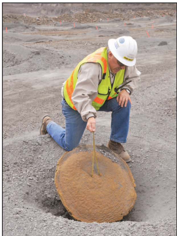
Indihar lifts the protective cover off a drilled blast hole. The covers are in place until charges are set in the hole then sealed with rock.
