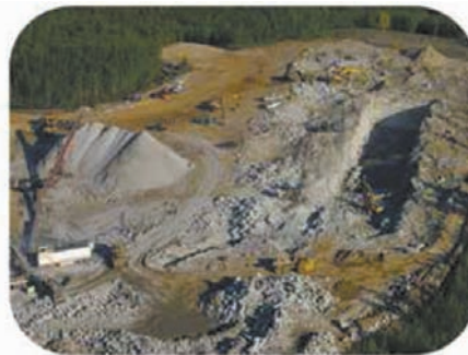
NoVA During Construction
