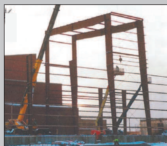
Magnetation, LLC Slon Building
