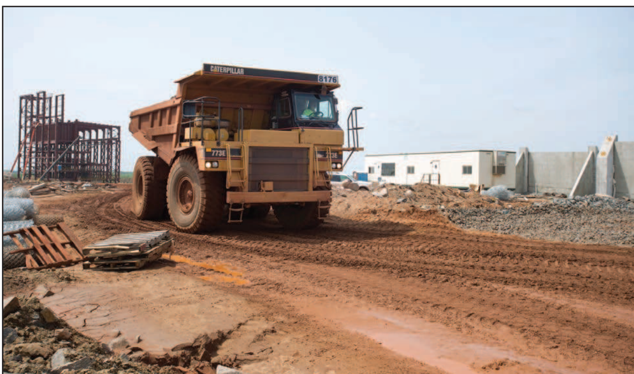
A truck hauls 60 tons of taconite ore to be used as fill around a processing building.
