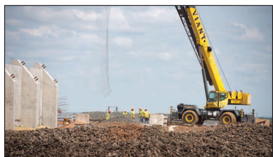
Fill rock is placed around an ore processing area.
