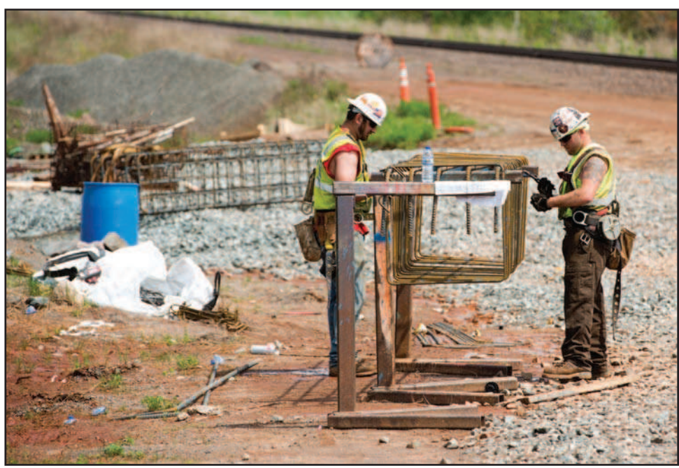
Workers shape rebar.
