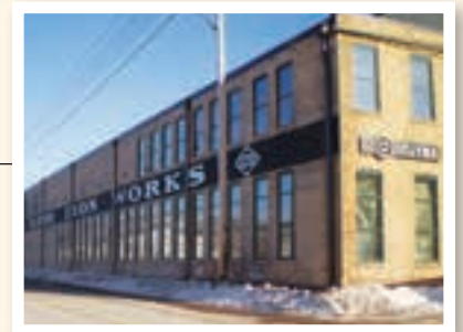
2010 – Clyde Iron Works renovation
