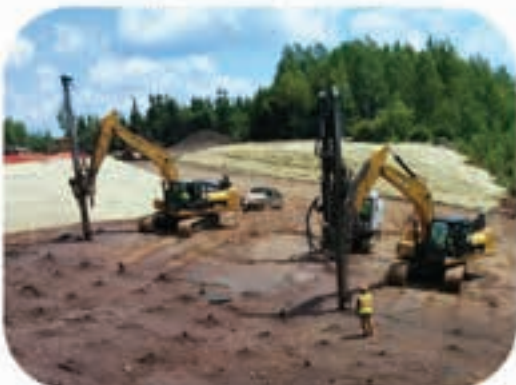
Hwy 53 Reroute Drilling and Blasting
