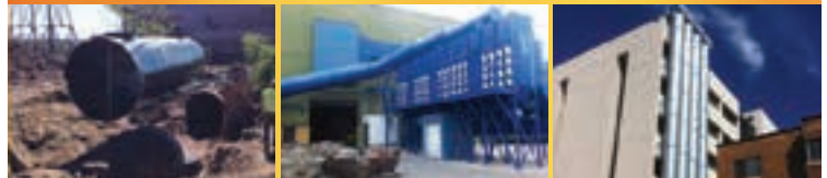
◆ Mill Water Line Replacement ◆ Dust Collection System ◆ Temporary Fresh Air Ductwork Installation
