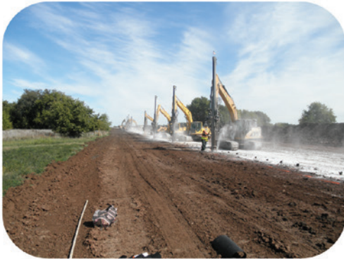
Flanagan South Pipeline Drilling and Blasting
