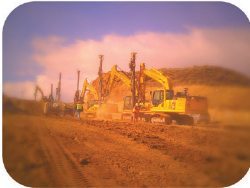
Ruby Pipeline Drilling and Blasting
