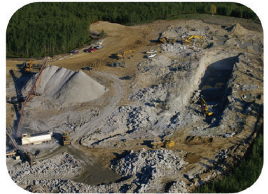
NOVA During Construction
