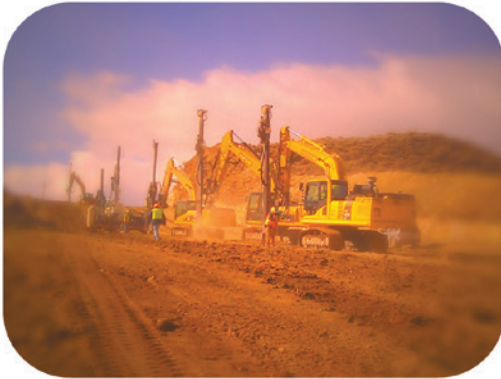
Ruby Pipeline Drilling and Blasting
