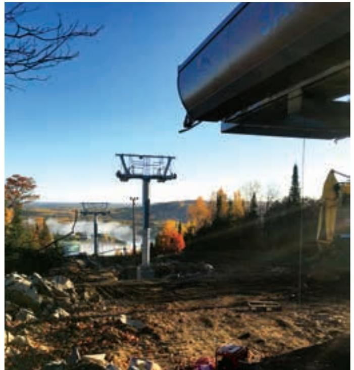
One of the biggest obstacles to overcome was the lack of any road access to the top of the hill. Lakehead built a road on the existing topsoil and pulled all of the lift components and equipment up the steep hill with bulldozers.
