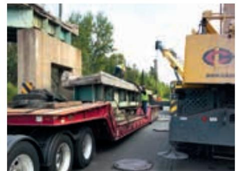
the concrete deck was done to expose the structural steel on both ends, and torches were used to slice through the steel, which was resting on concrete columns. Once this was accomplished, the lift could be made. The father-son team of Steve Levine, shop manager, and Jake Levine, crane operator, lifted and turned the 56-ton section smoothly to the ground parallel to the highway at precisely 7 a.m.
